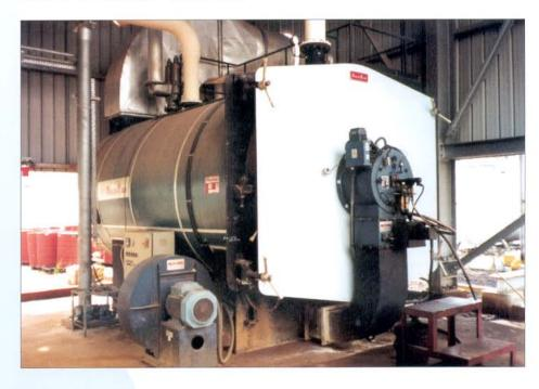
THE HT MODEL IS BUILT TO CONFORM TO BS2790 OR ANY OTHER INTERNATIONAL STANDARDS ON SPECIAL REQUEST.
