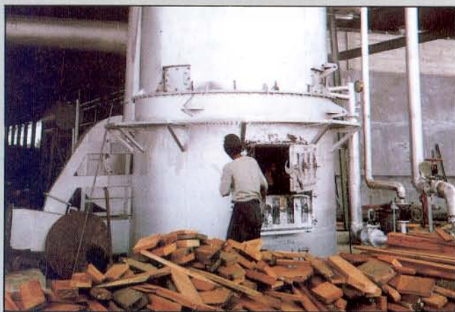
Complete unit of a 10 MBTU heater installed at site in Indonesia. Fuel being used is sawmill off-cuts.
